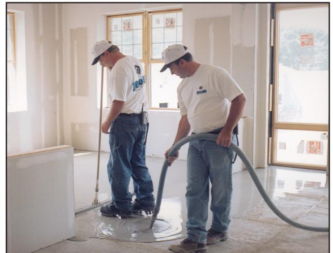
With the installation of FIRM-FILL Gypsum Concrete, Gypsum Floors, Inc. provided the resort with smooth, flat durable floor surfaces and upgraded sound control, ready for the installation of finished floor coverings.
