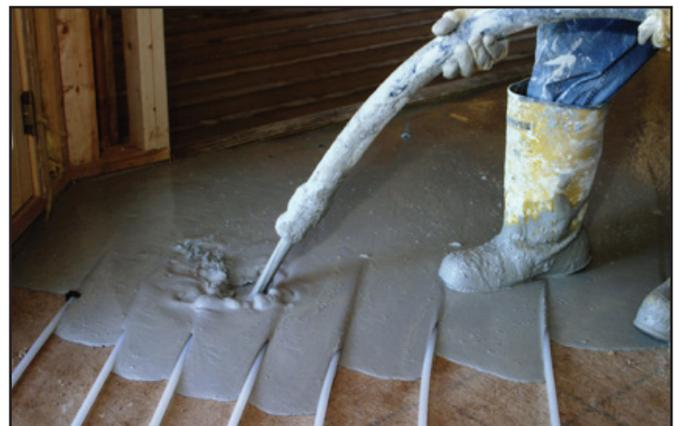
installed over the heat source, it seals the room's perimeter and adheres to the tubes or cables, spreading heat evenly throughout the floor without hot spots. **GYP-SPAN® Radiant** dries without shrinkage cracks and provides a smooth, flat, energy efficient thermal mass on which finished floor goods can be easily attached.
