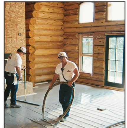
Hacker Industries, Inc. supplies an entire line of Firm-Fill® gypsum concrete floor underlayments that possess superior strength and ultimate sound control, with PSI strengths ranging from 1200 to over 5500. With over 105 Underwriters Laboratories listings, and ratings from ICBO, BOCA, SBCCI, and HUD, Firm-Fill®
