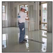
in conjunction with FIRM-FILL® Brand Gypsum Underlayments. FIRM-FILL® SCM can improve IIC ratings 15-25 points and carry a Class-A fire rating under ASTM E84.
