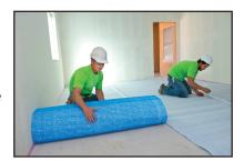
FIRM-FILL® SCM are the only sound control mats that are color coded for quality control. These durable, lightweight sound control mats are engineered to limit impact and airborne sound transmission between units when used
