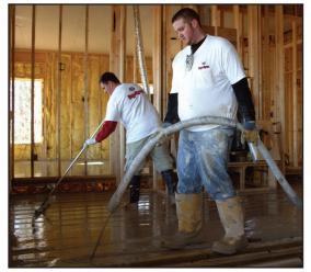
In the search for a product that would provide warm, comfortable floors and uniform heat, General Contractor Addco Builders selected **GYP-SPAN® Radiant** gypsum concrete floor underlayment. Known for its inherent high strength and energy efficiency, **GYP-SPAN® Radiant** provided a radiant heat system that ensured even heat transfer in every room.
