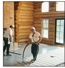
Hacker Industries, Inc. supplies an entire line of Firm-Fill® gypsum concrete floor underlayments that possess superior strength and ultimate sound control, with PSI strengths ranging from 1200 to over 5500. With over 105 Underwriters Laboratories listings, and ratings from ICBO, BOCA, SBCCI, and HUD, Firm-Fill®
